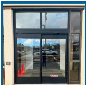
South Davis Installed February 2024
