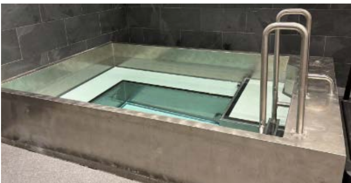
Cold plunge pool after completion
