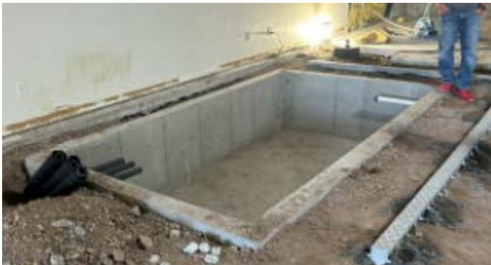
Cold plunge pool during construction
