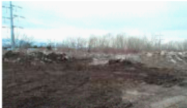
DURING DEBRIS REMOVAL
